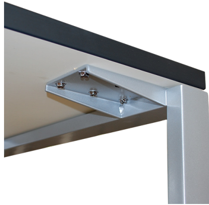
Detail: base placement
